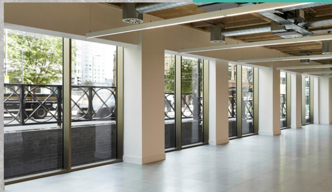
THE REFURBISHMENT INCLUDES NEW FLOOR-BY-FLOOR VRF AIR CONDITIONING WITH A NEW AIR HANDLING SYSTEM FOR OPTIMUM PERFORMANCE. EXPOSED SERVICES MAXIMISE THE FLOOR-TO-CEILING HEIGHT ALBEIT THIS CAN BE ADAPTED TO SUIT REQUIREMENTS.
